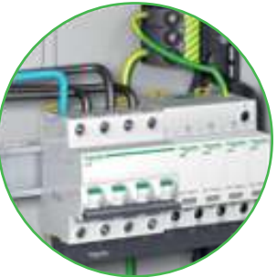
Surge arrester iPRD 4P + iC60N 4P
